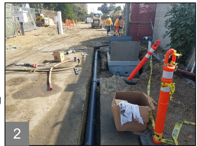
Photo 2 – Installing SVE pipe (looking east along ROW)
