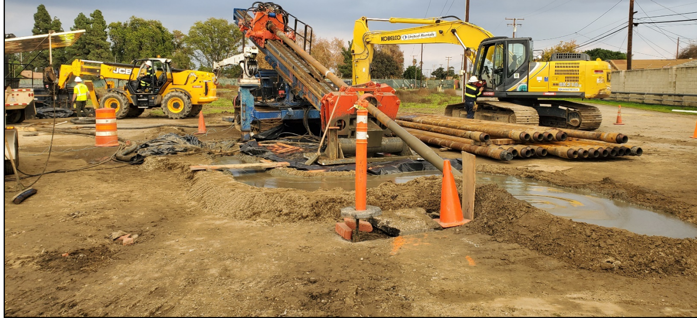
Photo 1 – Drilling the Horizontal SVE Well
