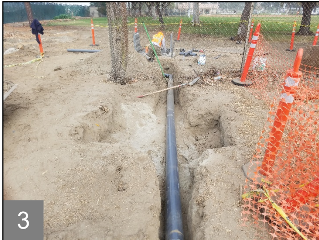
Photo 3 – Installing SVE pipe (looking north towards Holifield Park)
