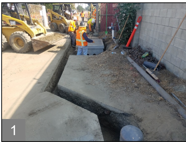
Photo 1 – Trenching SVE lines (looking east along ROW)
